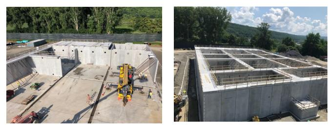
In 2019, Dutchland built a precast post-tensioned SBR tank at the Village of Watkins Glen WWTP in Schuyler County, NY. Previously, the Villages of Watkins Glen and Montour Falls each operated aging municipal wastewater treatment plants. The two villages jointly developed the new WWTP and decommissioned their respective facilities when the new plant was operational.
