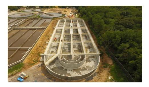
**Description**: In order to meet the needs of a growing community, the Patuxent WRF began an expansion project to increase the capacity of the plant from 7.5 MGD to 11.6 MGD. The project scope included a new headworks facility, influent pumping station, third oxidation ditch, fourth clarifier, and denitrification filters. The commissioning for the project was required by October 2018 so that developers could tie-in to the Patuxent Sewershed.
