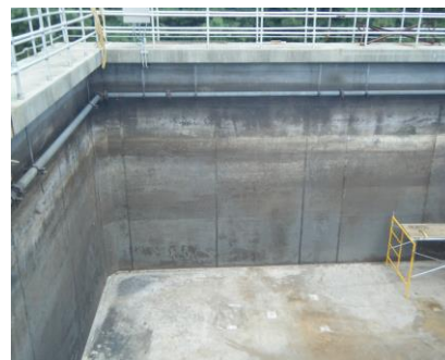
Photo taken after original SBR built in 1991 was pumped down on 8/9/10.
