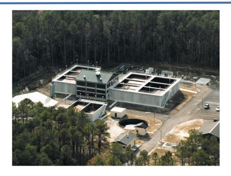
Capacity: 1.4 MGD Sequencing Batch Reactor and Equalization Tank
