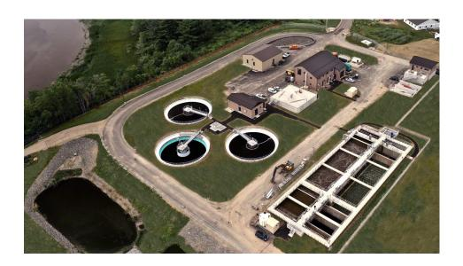
**Background:** The Exeter WWTF has a design average capacity of 3 MGD, with a peak flow capacity of 7.5 MGD. The WWTF was constructed in 1965 and was upgraded in 1990 (lagoon expansion) and in 2002 (outfall upgrade).
