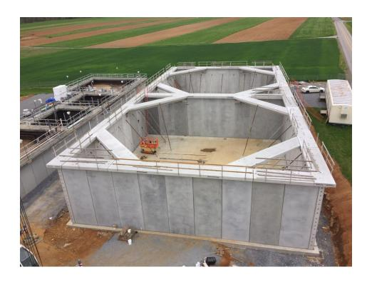
**Description**: In 1995, Dutchland designed and constructed a wastewater treatment plant with an average daily flow of 0.48 MGD for Earl Township to serve the Gardenspot Village Retirement Community. The tank footprint measures 154′-2″ long by 47′-8″ wide by 21′ tall and consists of a two-basin SBR, dual digesters, and a post-equalization tank under the control building.
