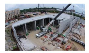
Capacity: 18 MG rectangular CSO tank Structure Footprint: 415-ft by 256-ft On-site Project Duration: 10 months Total Precast Concrete Pieces: 1,733
